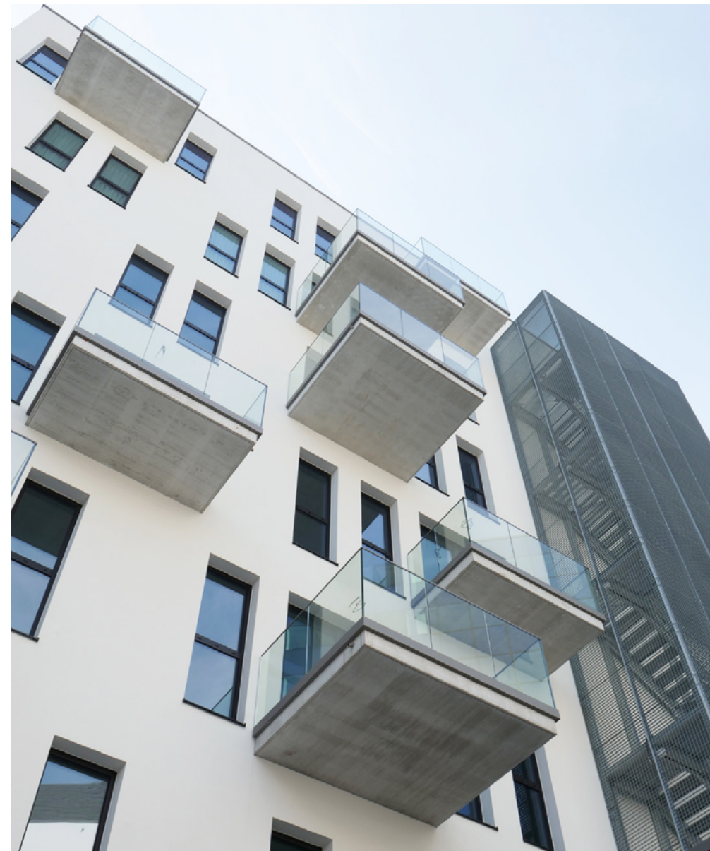
The new Hôtel ibis Styles Liège Guillemins in Belgium is a 102-bedroom modern 3 star hotel with a unique and fun comic book themed interior decorative concept throughout. Prefaco, part of CRH's Europe Materials Division provided a range of precast concrete solutions to the project including 16,000 m 2 shuttering slabs, 10,000 m 2 double walls, 30 m 3 beams and 102 stairs.
