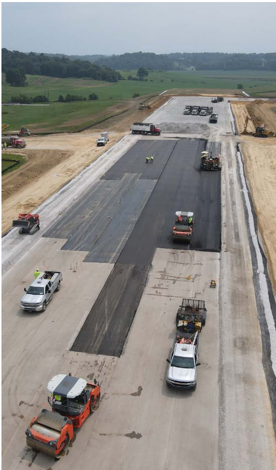
J.H. Rudolph & Co., Inc, part of CRH's America's Materials Division, delivered this runway extension project at Huntingburg Regional Airport in Indiana, United States. The project included increasing the length of the runway by over 500 feet and the construction of Indiana's first traffic tunnel under an airport runway.
