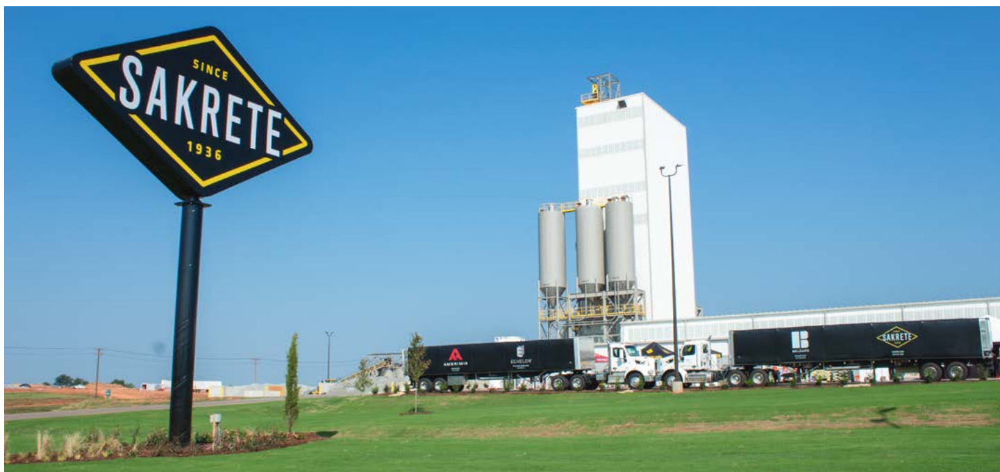
In 2021 Oldcastle APG, part of CRH's Building Products Division, opened a new dualbagging-line, dry-mix facility located at Cowpens, South Carolina, United States. The plant's high throughput capability and strategic geographic location between Charlotte and Atlanta, the fastest growing population centers in the southern United States, bolsters APG's end-to-end solutions offerings for customers in the region.
