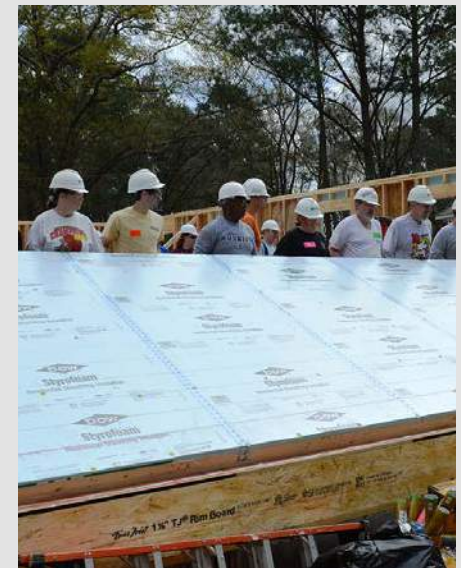
Volunteers working on an Oldcastle, Habitat for Humanity build.
