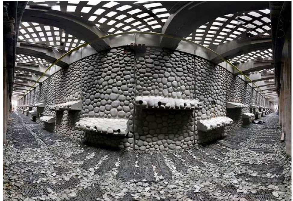
CRH Company, Oldcastle Precast supplied the concrete Z-superstructure segments, sidewalk panels and face panels for the upgrading of the Elliott Bay Seawall. Originally built in the 1850s, the seawall was at risk of deterioration and collapse before the project revitalised the waterfront area in downtown Seattle, Washington, US by shoring up infrastructure, providing pedestrian access to the water and creating a safe habitat for marine life including migratory salmon.
