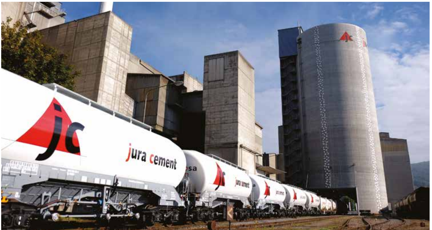
Rail transport of bulk cement at Jura Cement's Wildeggen plant in Switzerland. Jura uses 75% alternative fuels and produces ECO JURA cement, which has an eco-label for its lower carbon footprint.
