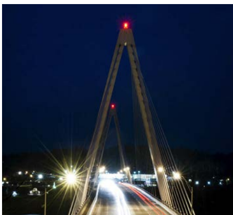
The Shelly Company's Smith Concrete supplied 35,000 cubic yards of concrete for the US$45 million Bridge of Honor. The bridge is a cast-in-place segmental concrete edge girder system with transverse floor beams. The bridge, which has a span of 675-feet, connects the cities of Pomeroy, Ohio, and Mason, West Virginia, across the Ohio River.
