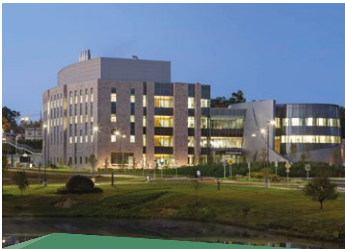
Featuring 44,000 square feet of Reliance™-TC type II curtain wall from Oldcastle BuildingEnvelope®, the Jackson Laboratory for Genomic Medicine, Farmington, Connecticut, US is a prominent LEED®-certified, Gold rated project. The entire curtain wall was custom-engineered for maximum thermal performance.
