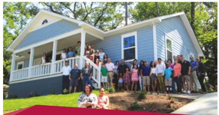
More than 250 employees and their families and friends volunteered on the 4 th Oldcastle Habitat for Humanity Home which was constructed in Atlanta, Georgia, US in 2014. Oldcastle donated materials such as blocks and mortar, retaining walls, siding, countertops, pavers and roofing materials.
