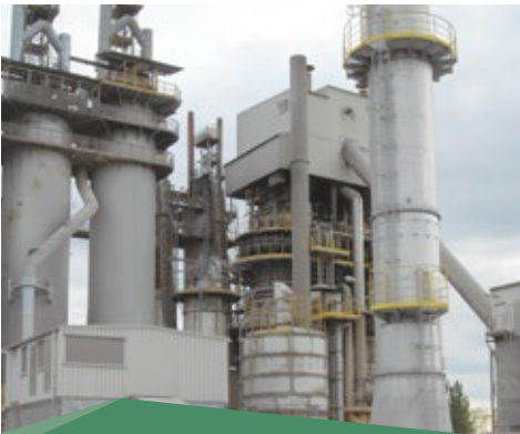
Trzuskawica Lime upgraded the dedusting installation at its lime plant in Sitkówka, Poland, to abate particulate emissions.
